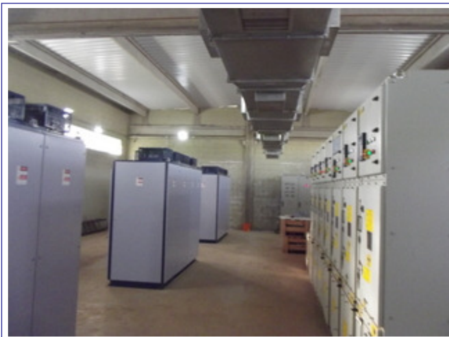
SUBSTATION / CCM GRINDING
