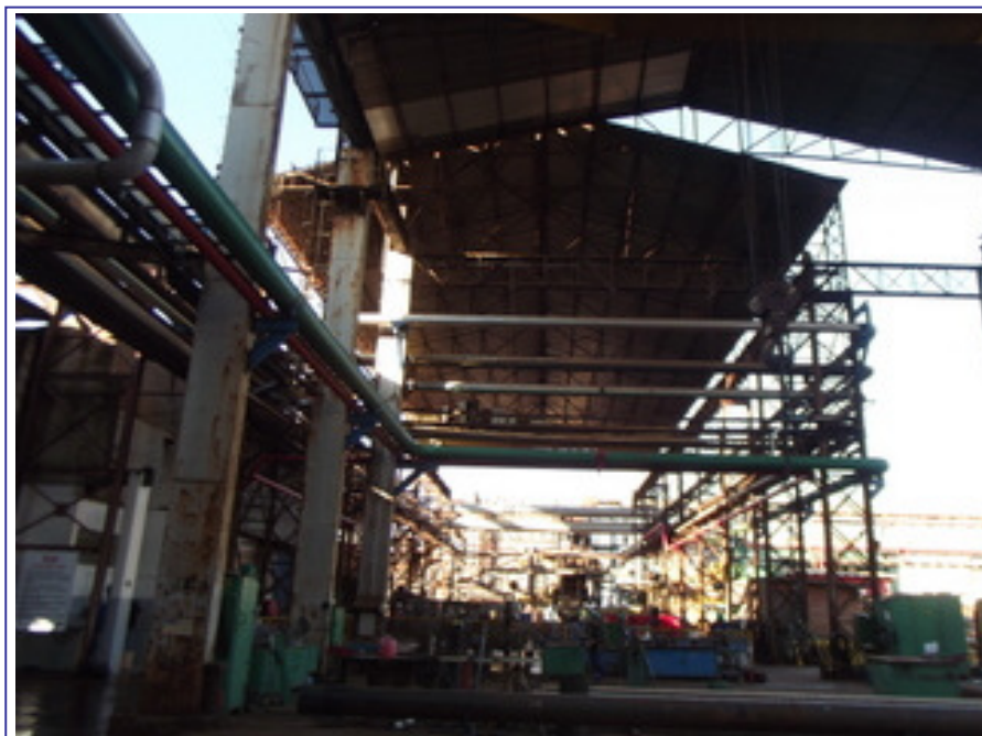
NON-USED GRINDING EQUIPMENT
