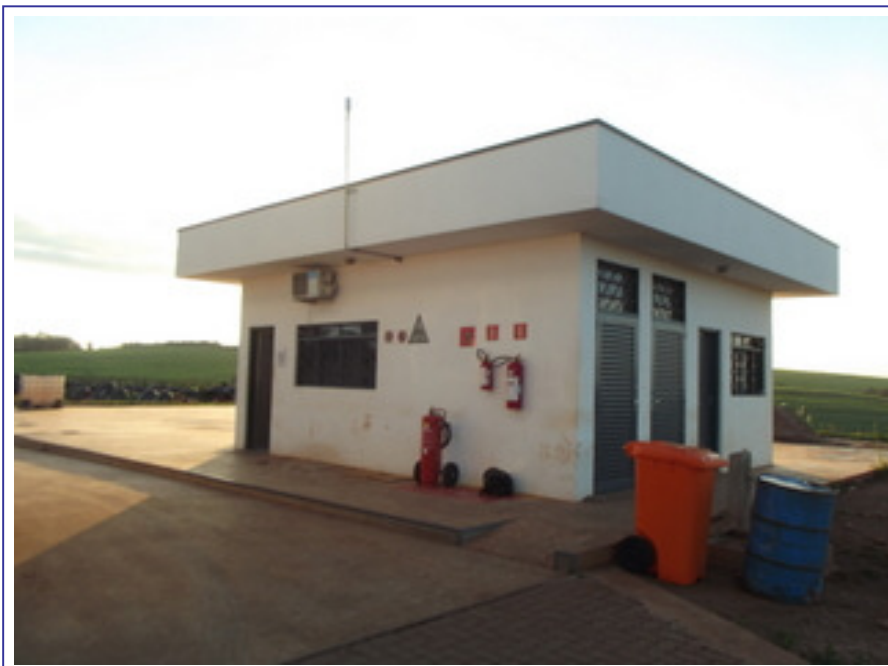
SUPPORT TO FUEL STATION
