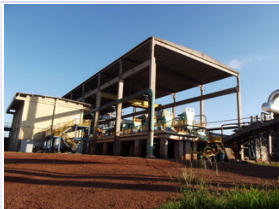
CCM STATION & GRINDING EQUIPMENT
