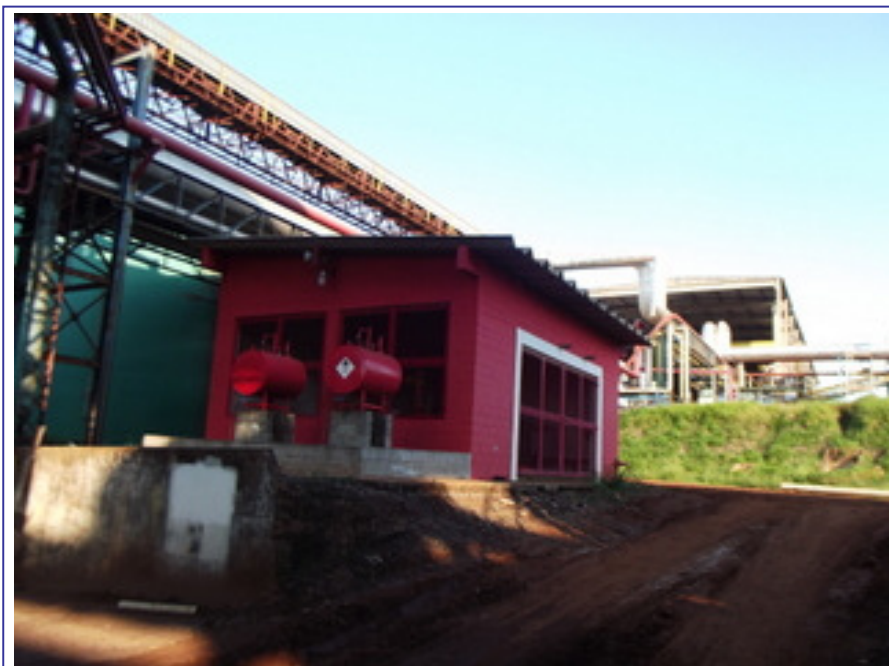
FIRE PUMP ROOM
