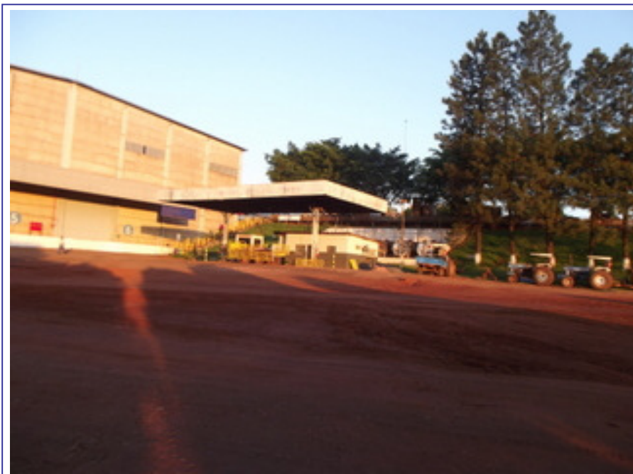
NON-USED FUEL STATION
