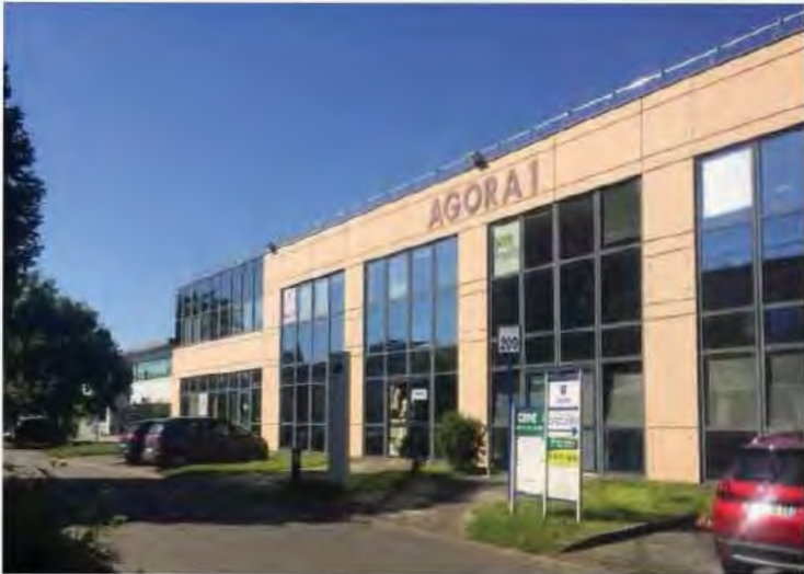
Exterior view building 2
