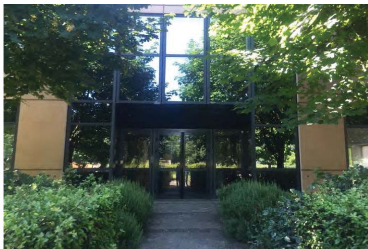
Exterior view building 1
