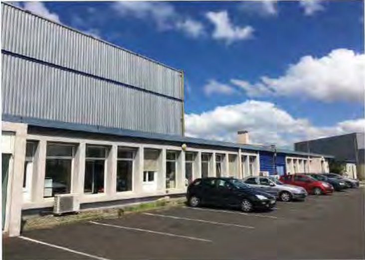
View of the office building
