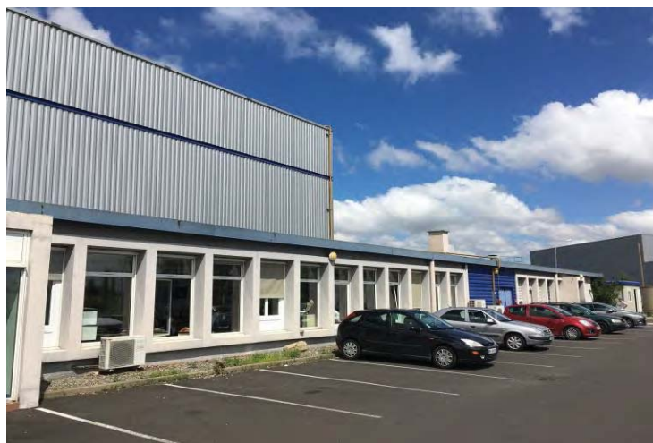
View of the office building
