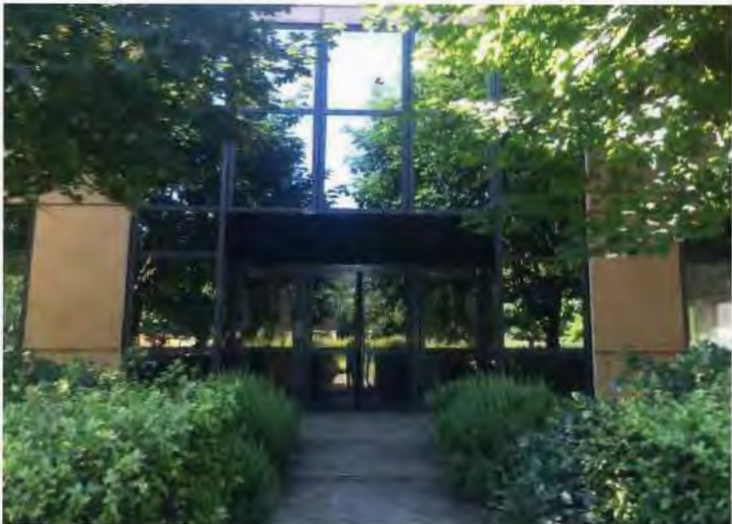
Exterior view building 1
